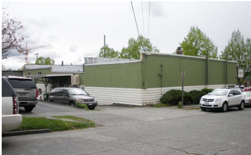
3 VIEW OF SITE FROM THE NORTHEAST
