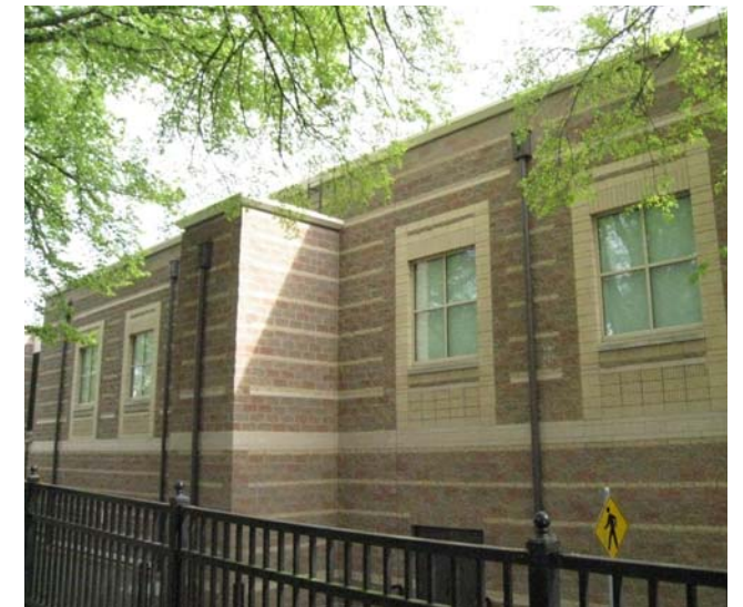
Roosevelt Highschool Addition Interesting use of building masonry which relates to the original high school without trying to copy the original detailing. The horizontal banding and oversized suggested window frames provides a traditional character in a newer material.
