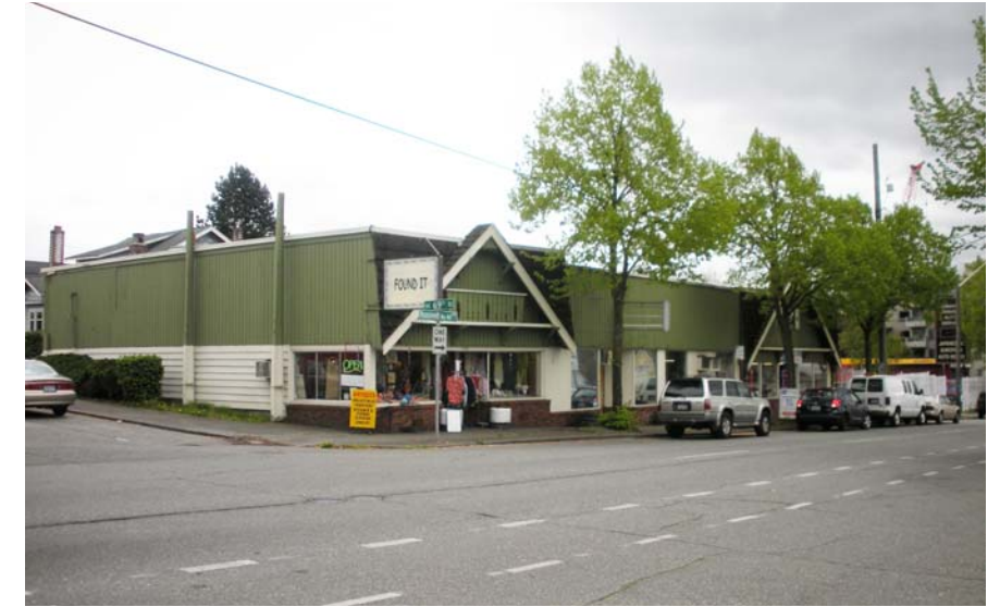
2 VIEW OF SITE FROM THE NORTHWEST
