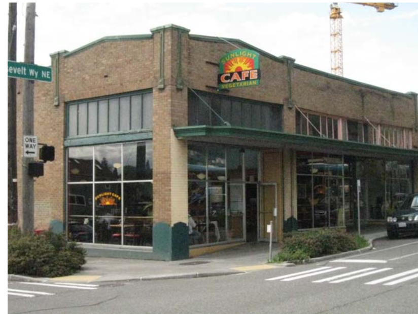
Sunlight Cafe 6403 Roosevelt Way NE Common 1.5 story traditional retail shops buildings along Roosevelt Way
