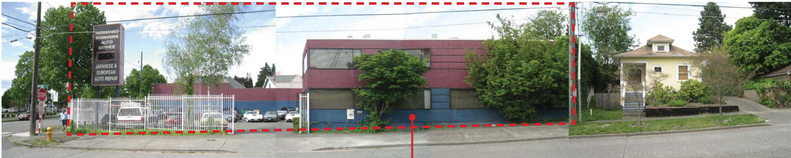
② NE 68th Street - North Side
