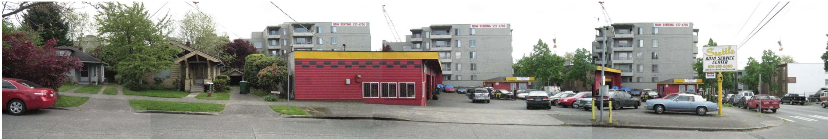
② NE 68th Street - South Side
