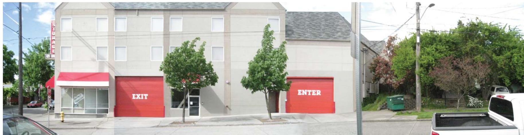
③ NE 69th Street - North Side
