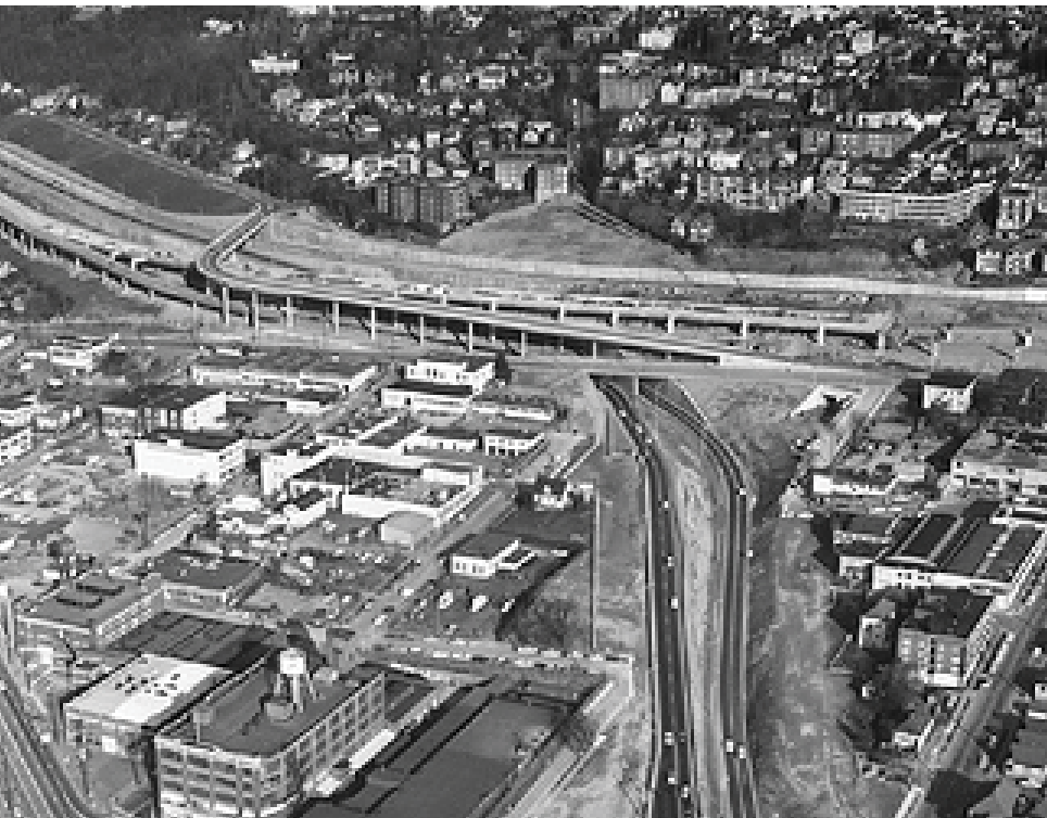
CIRCA 1965 AERIAL OF FREEWAY CONSTRUCTION SHOWING SITE (PHOTO SOURCE UNKNOWN)
