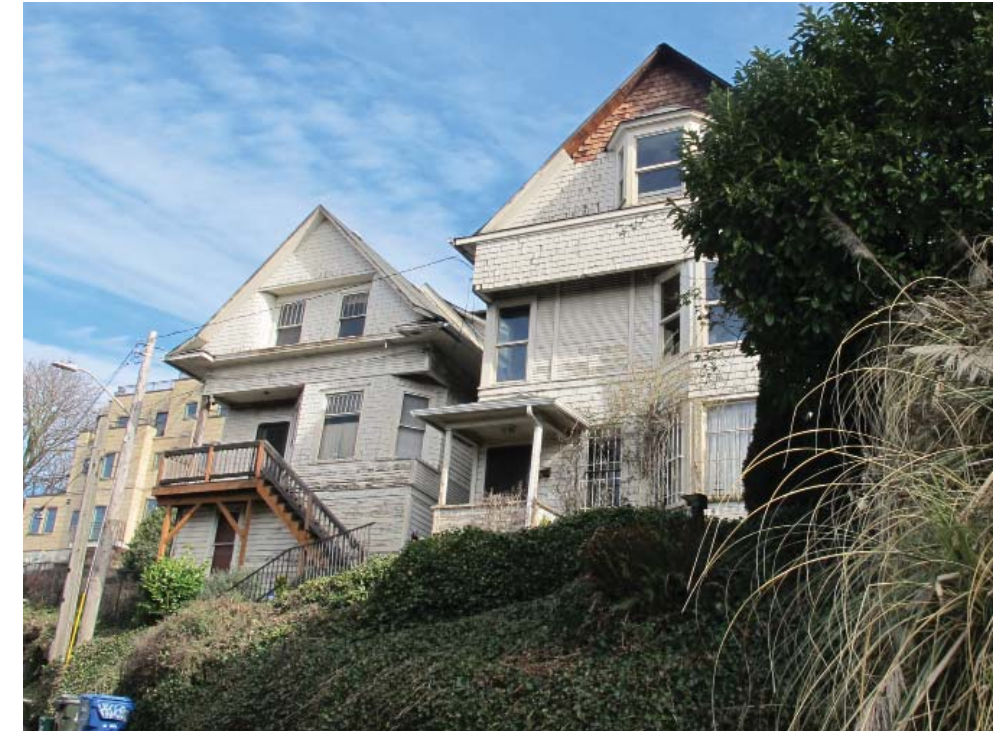
③ VIEW OF SITE FROM STREET
