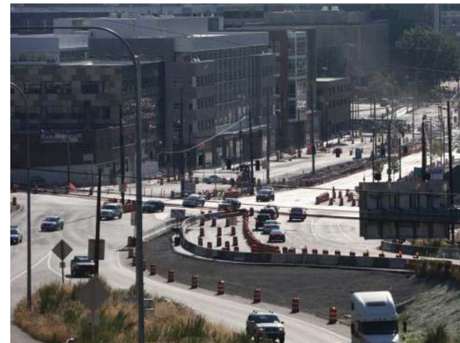
⑩ MERCER ON AND OFF RAMP
