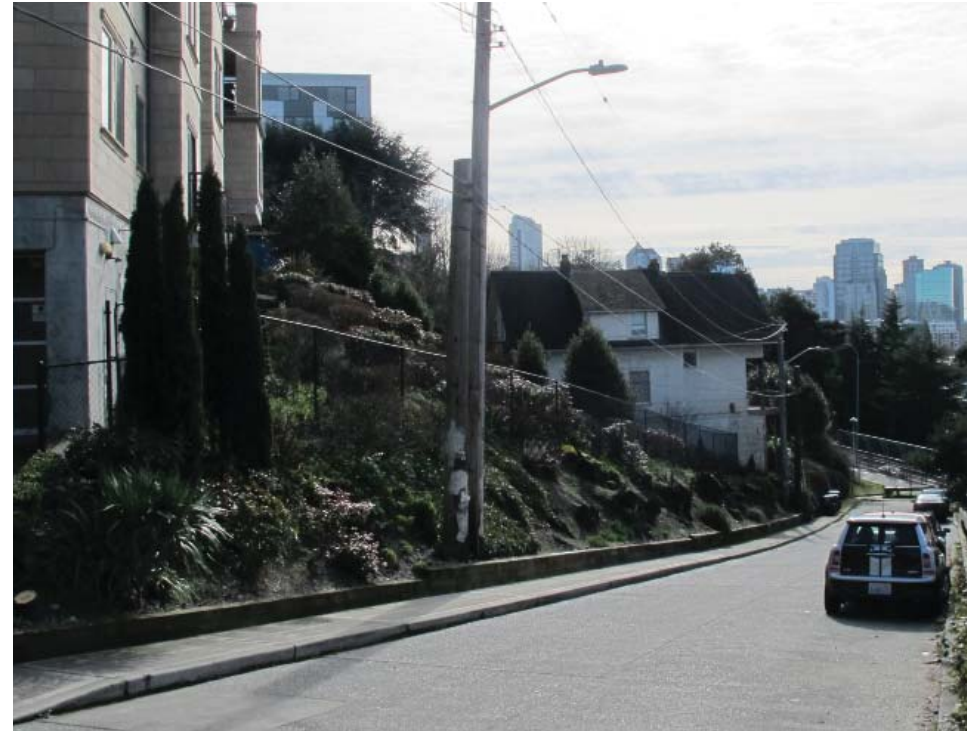
② VIEW OF SITE LOOKING DOWN BELLEVUE PLACE EAST
