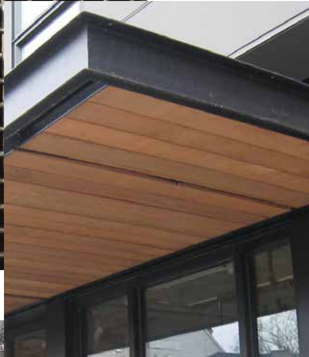
Steel awning with cedar soffit
