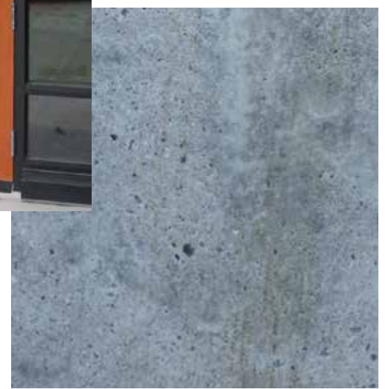
cast-in-place concrete garage walls @ site interior
