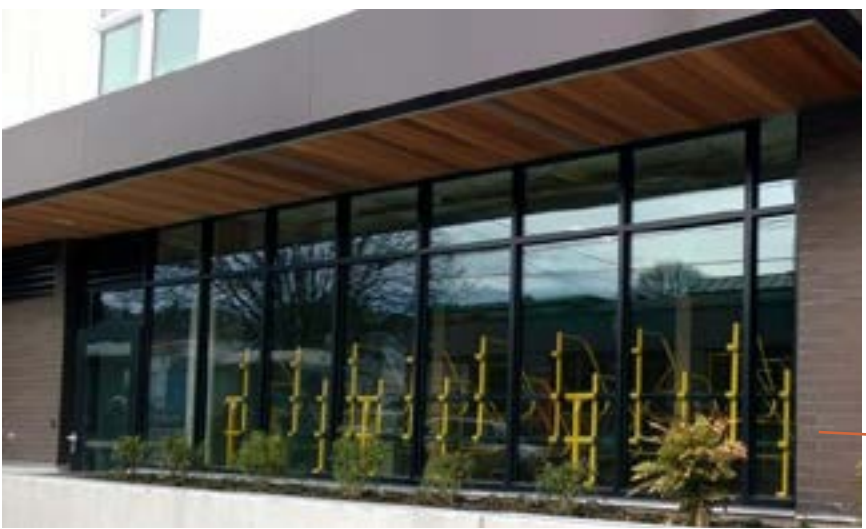
STREET-ORIENTED BICYCLE ROOM AT A PREVIOUS LAKE UNION PARTNERS PROJECT IN PORTLAND, OR
