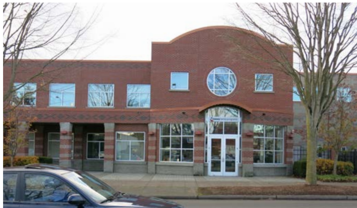
Large pedestrian-oriented storefront windows; durable building materials
