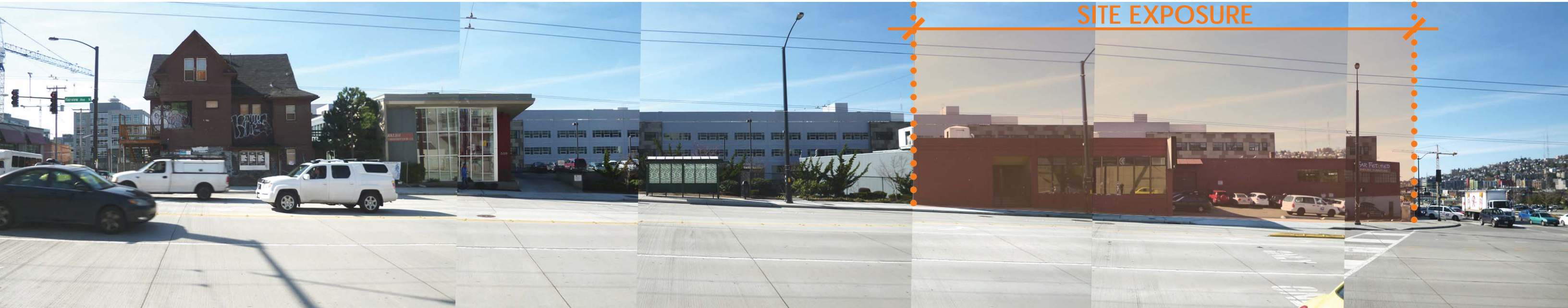
1 VIEW OF STREETSCAPE ALONG FAIRVIEW AVENUE N
