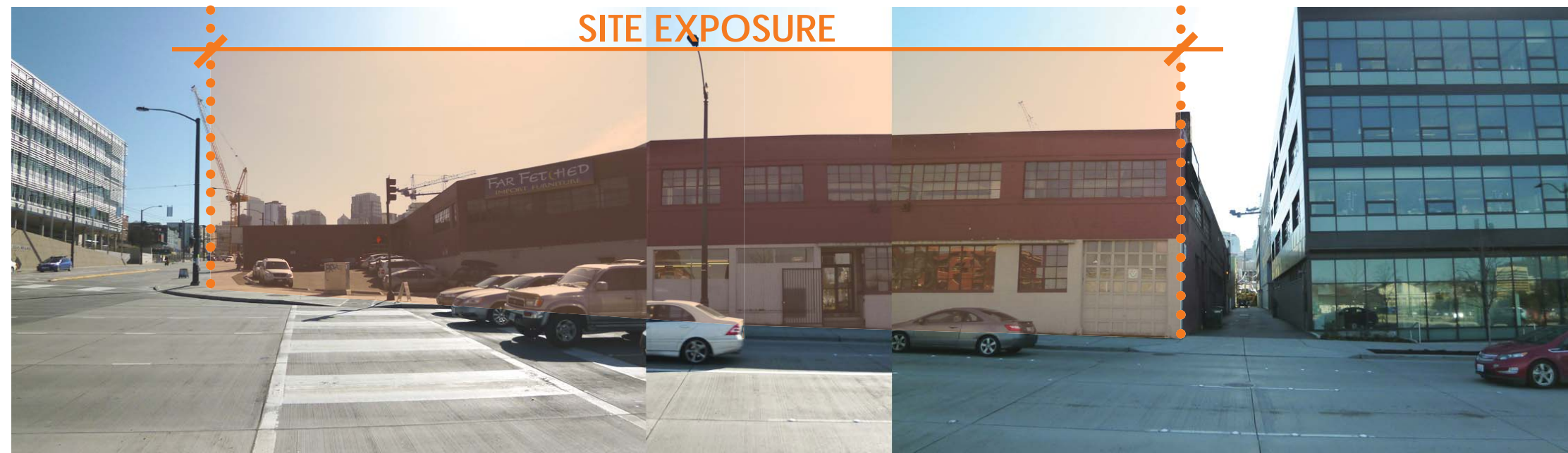
2 VIEW OF STREETSCAPE ALONG MERCER STREET
