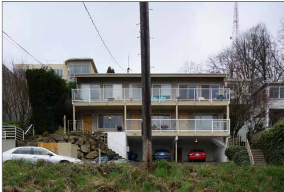
8 Entry stairs at 1243 5th Ave N
