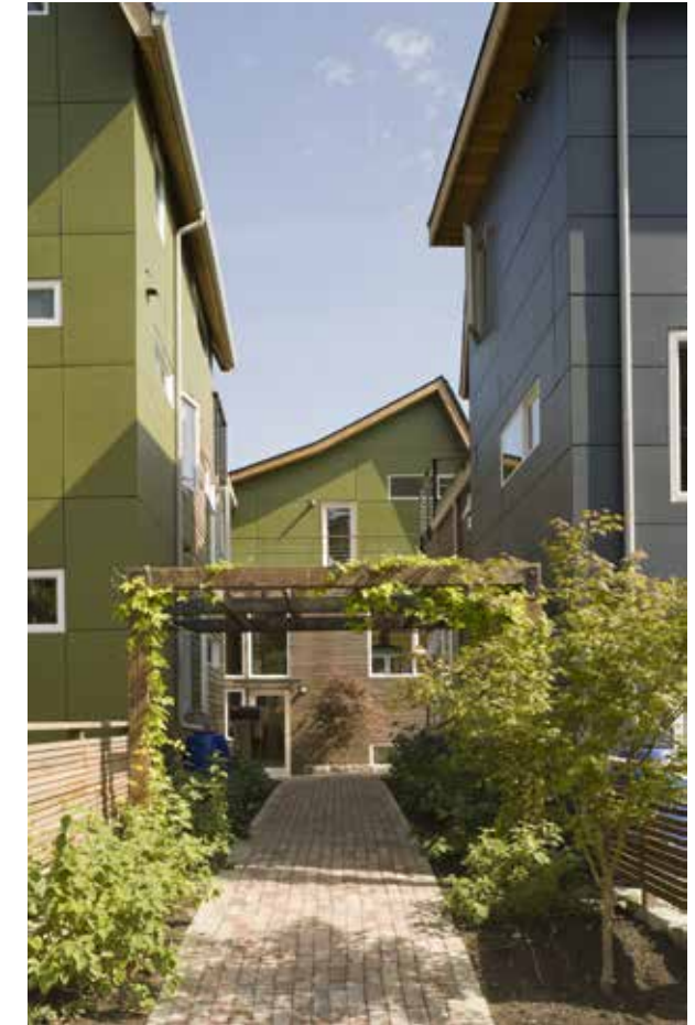
⑧ 1911 E. Pine St. view from street
