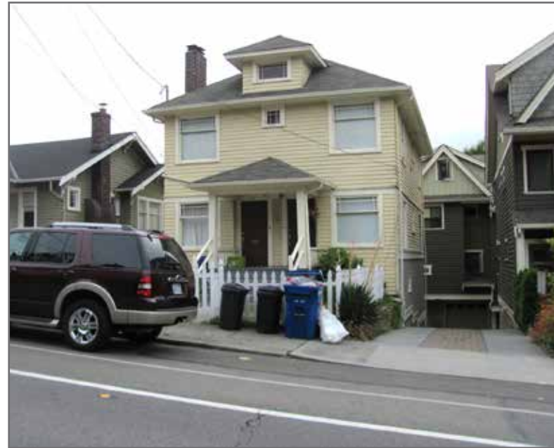
① Multi- unit entry at 1112 Taylor
