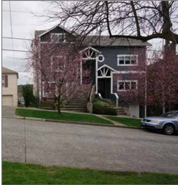
6 Entry stairs at 1218 5th Ave N.
