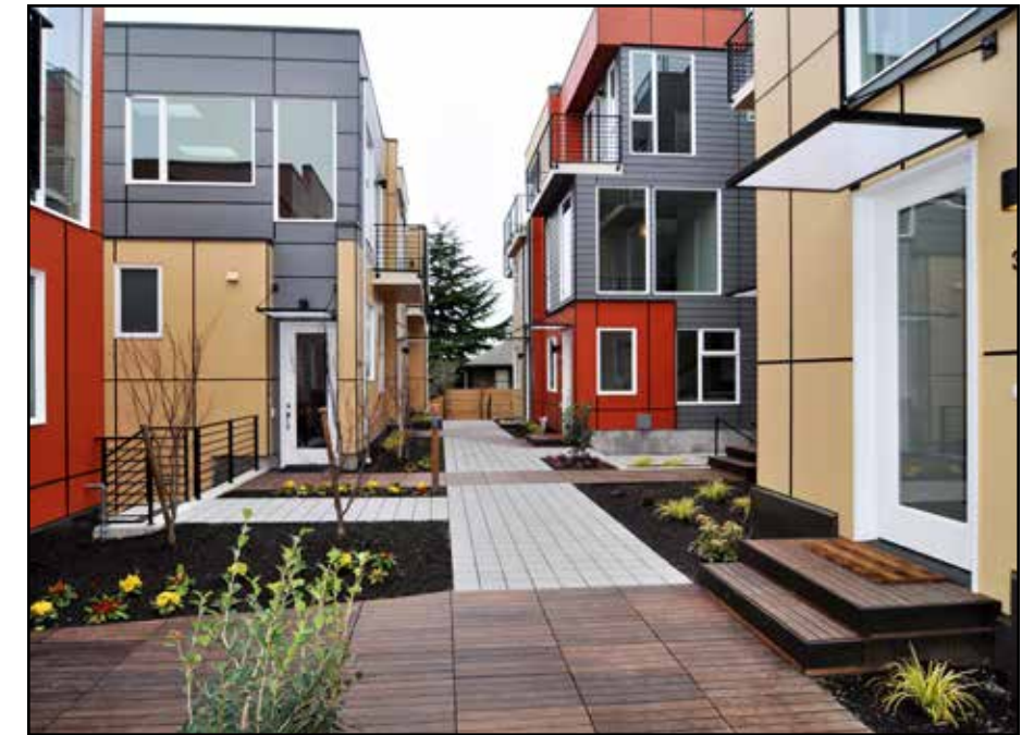
3515-3519 Wallingford Ave N courtyard view
