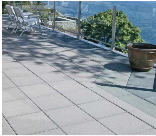
Pedestal Paver over structure
