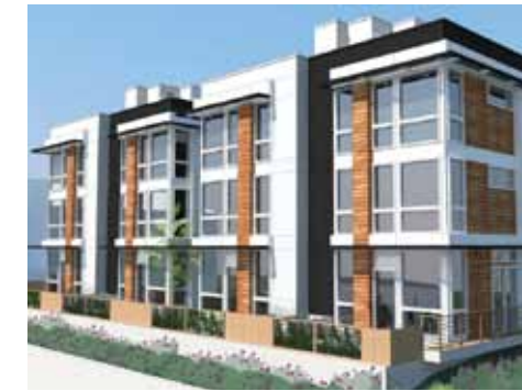
② TOWNHOMES - 4447 41ST AVE SW (UNDER CONSTRUCTION)
