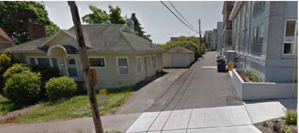
⑮ LOOKING SOUTH DOWN THE ALLEY FROM SW OREGON ST
