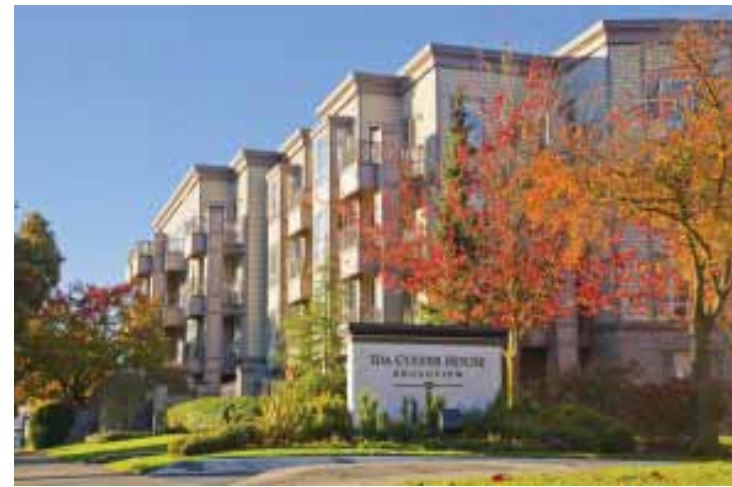
IDA CULVER HOUSE - BROADVIEW - SEATTLE, WA
