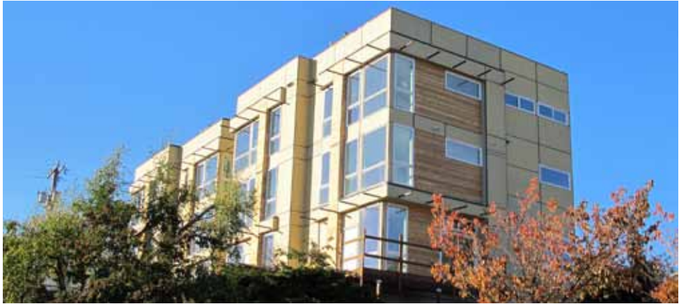
⑧ LOOKING NW ALONG 41ST
