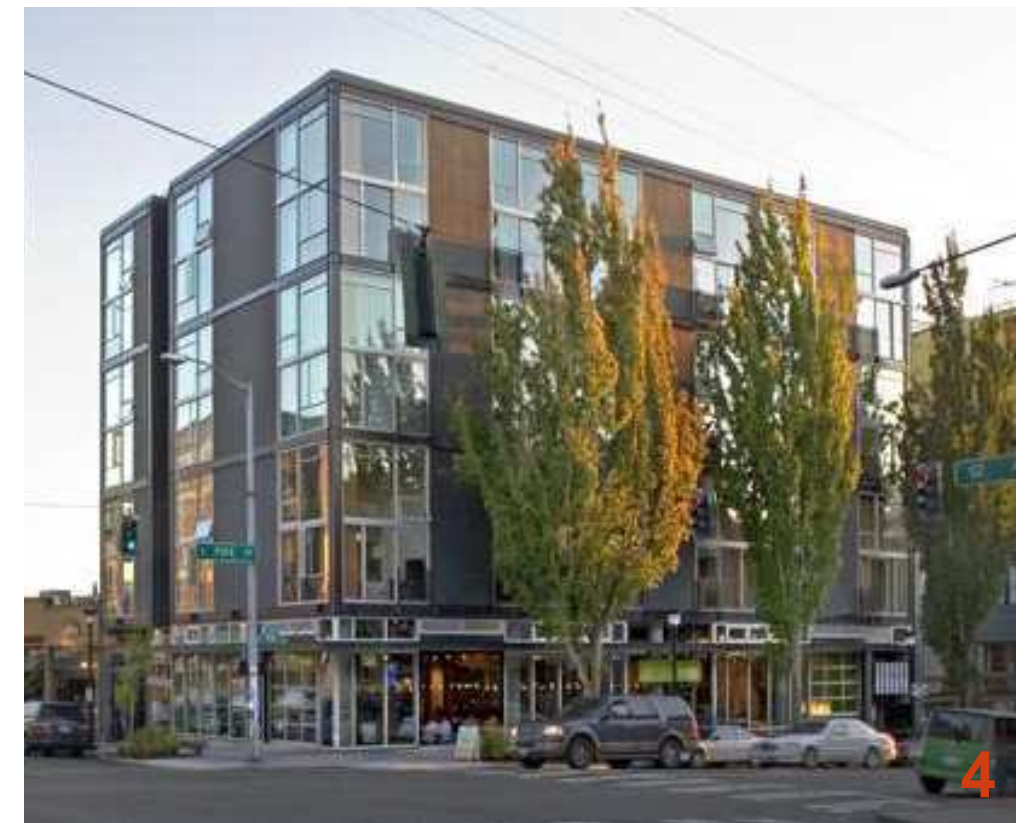
Agnes Lofts - Limited number of exterior finish materials. Simple and consistent fenestration.
