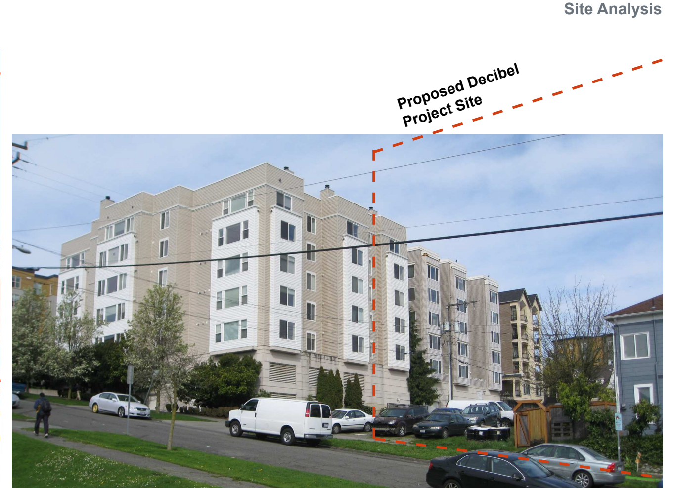
2 View of existing building to the west
