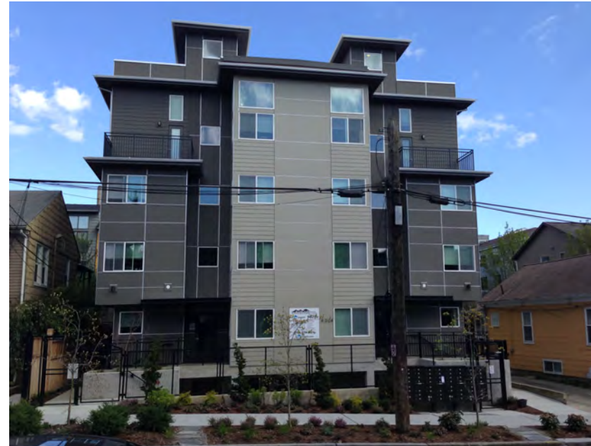
4324 8TH - ADJACENT PROPERTY TO THE NORTH DESIGNED BY ecco design inc.
