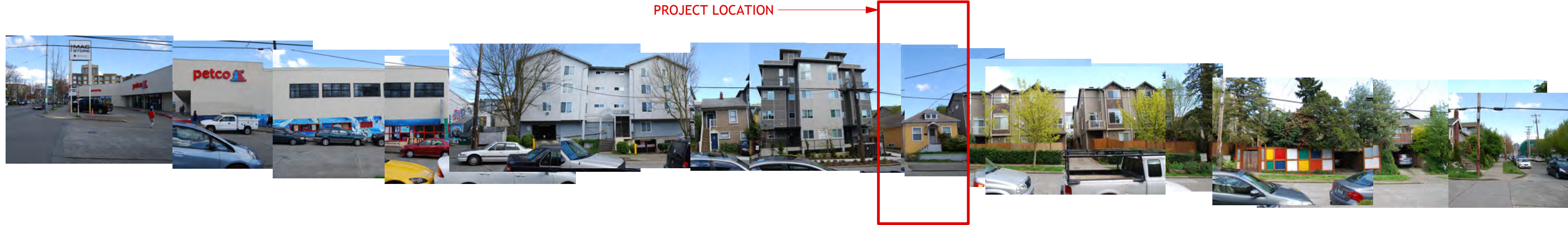
8TH AVENUE NE ELEVATION Looking east
