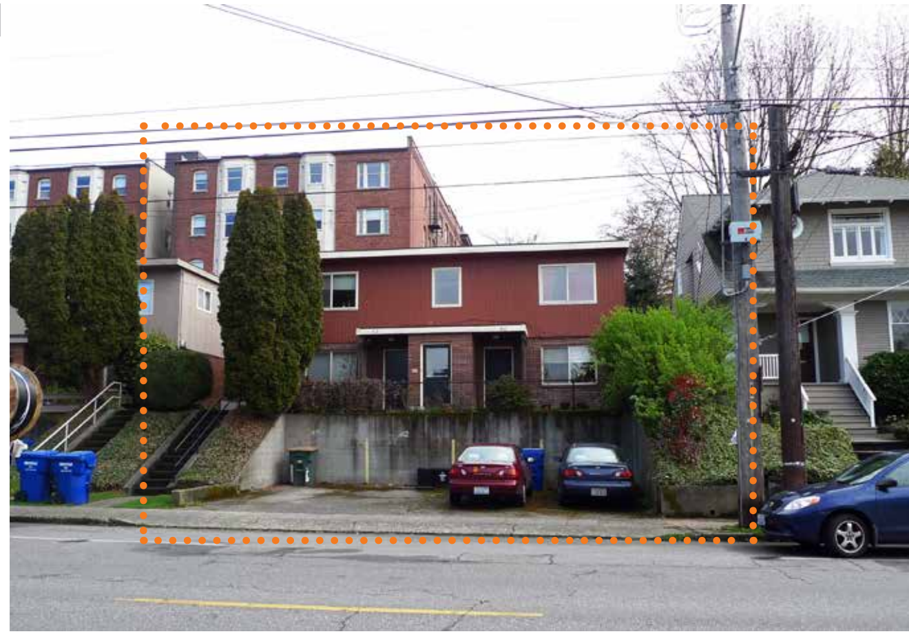
Project Site, existing single family structure to be deconstructed.
