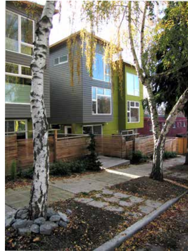
③ 1411 E. Fir St. exterior view from street
