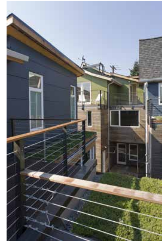
④ 1911 E. Pine St. courtyard view from a deck
