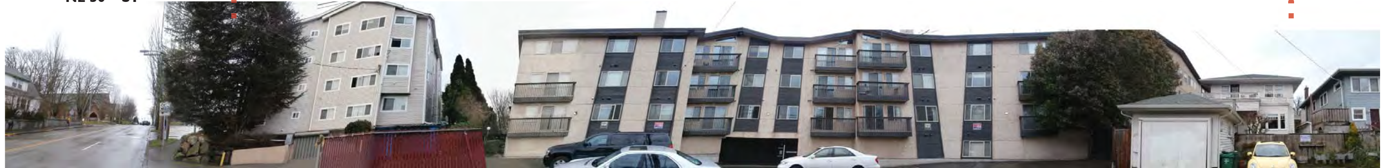
5 ADJACENT ALLEY LOOKING EAST - ACROSS FROM SITE
