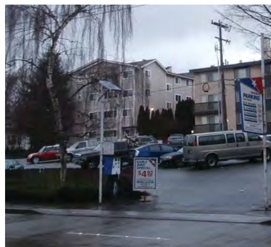
3 Existing curb cut to commercial parking lot mid block of site
