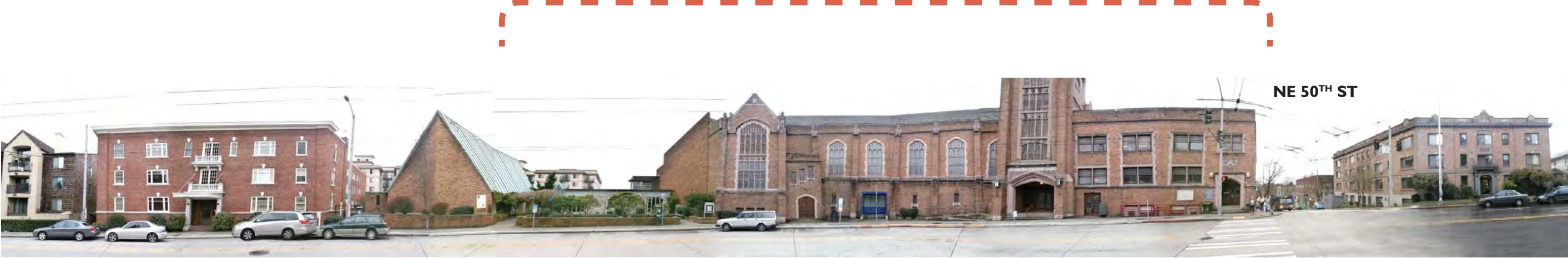
1 15 TH AVE NE LOOKING WEST - ACROSS STREET FROM SITE
