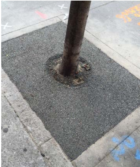
4 Flexi-pave Surfacing (At tree pit locations)
