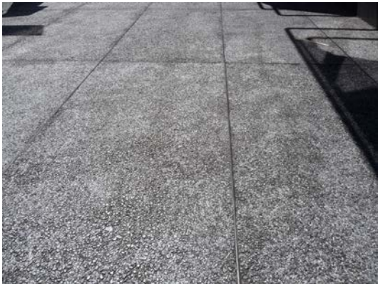
2 Top-seeded Aggregate Concrete Paving with Screed at Joints. Sidewalk to match existing at 2nd Avenue.
