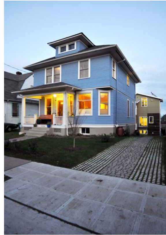
② 1504 19th Avenue Duplex behind SF House
