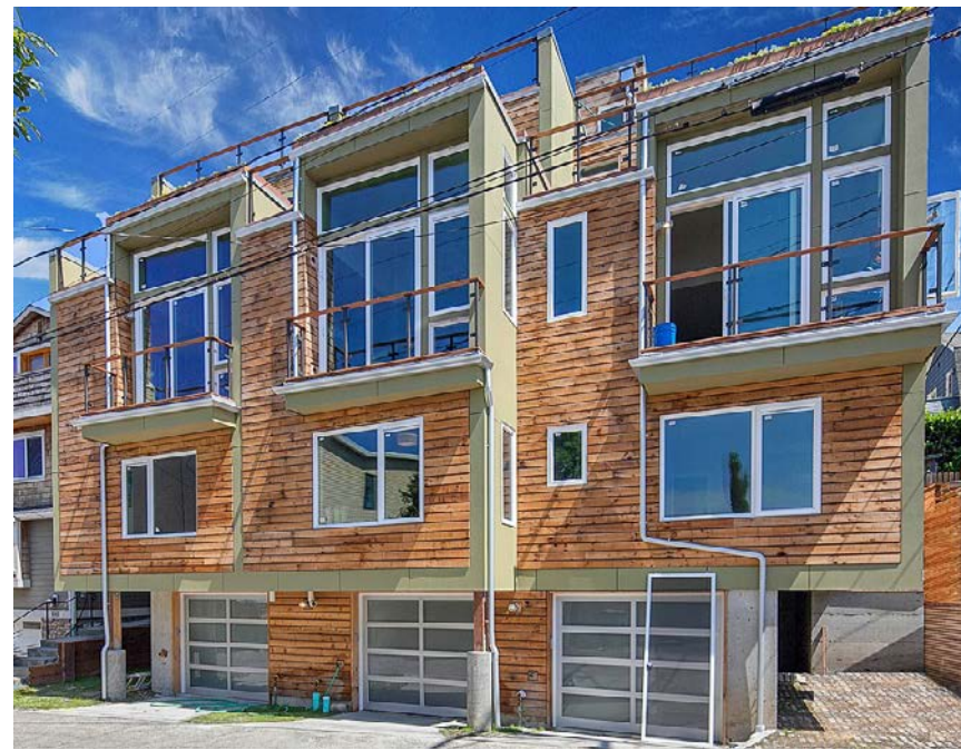
⑥ 1911 19th Ave W, view of alley facade
