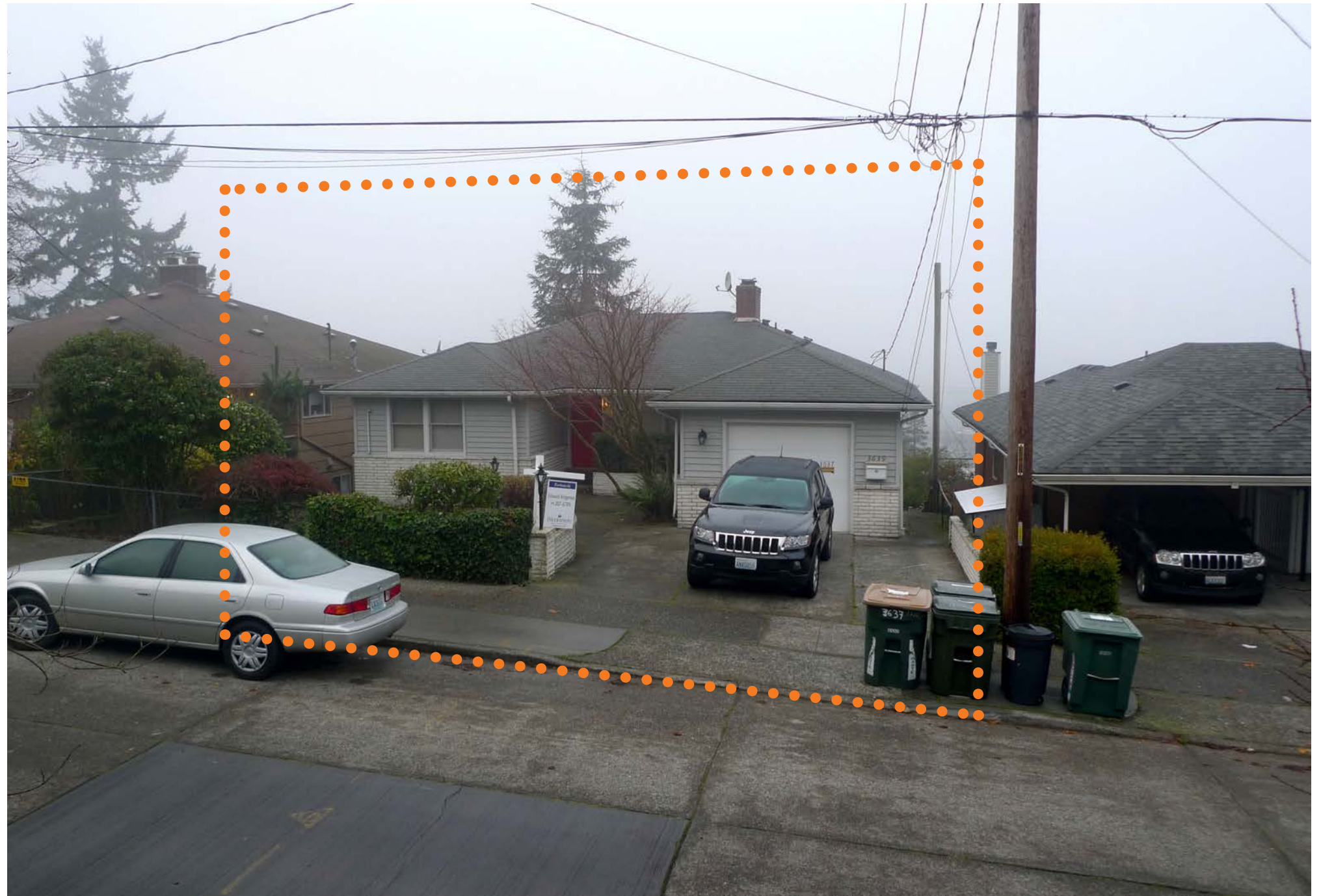
Project Site, existing structure
