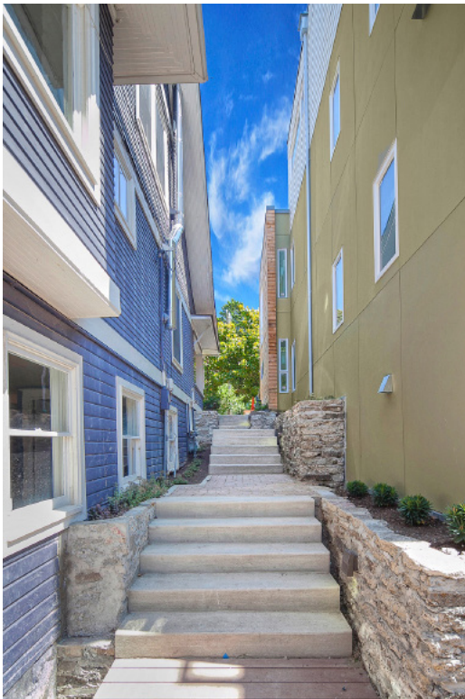
③ 1911 9th Ave W. view of entry walk
