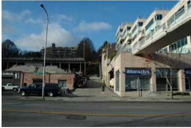
VIEW LOOKING WEST AT GALER ST
