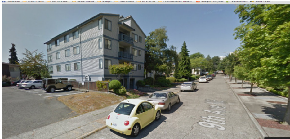
7. Neighboring Apartment Building
