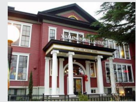
1 WALLINGFORD CENTER N 45TH ST AND BURKE AVE N HISTORIC COMMERCIAL SPACE IN WALLINGFORD
