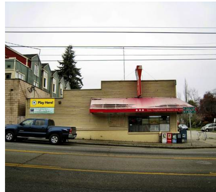
2 LOOKING NORTH AT PROJECT SITE FROM N. 50TH ST
