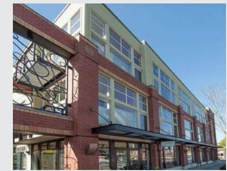
2 N 45TH ST & BAGLEY AVE N BRICK GROUND LEVEL WITH COMMERCIAL
