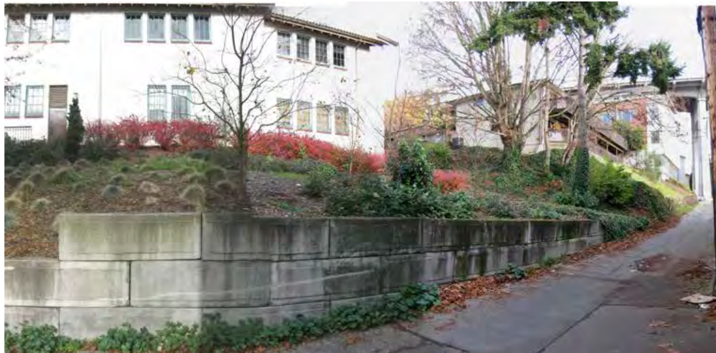
⑤ View of alley looking northeast
