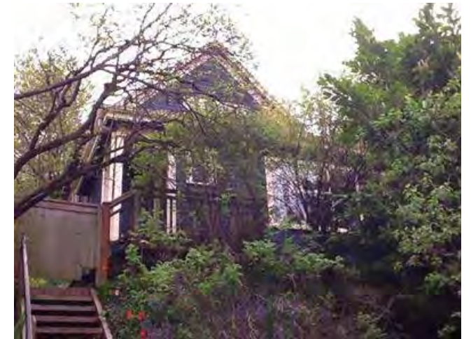
① Single family home on N 35th St
