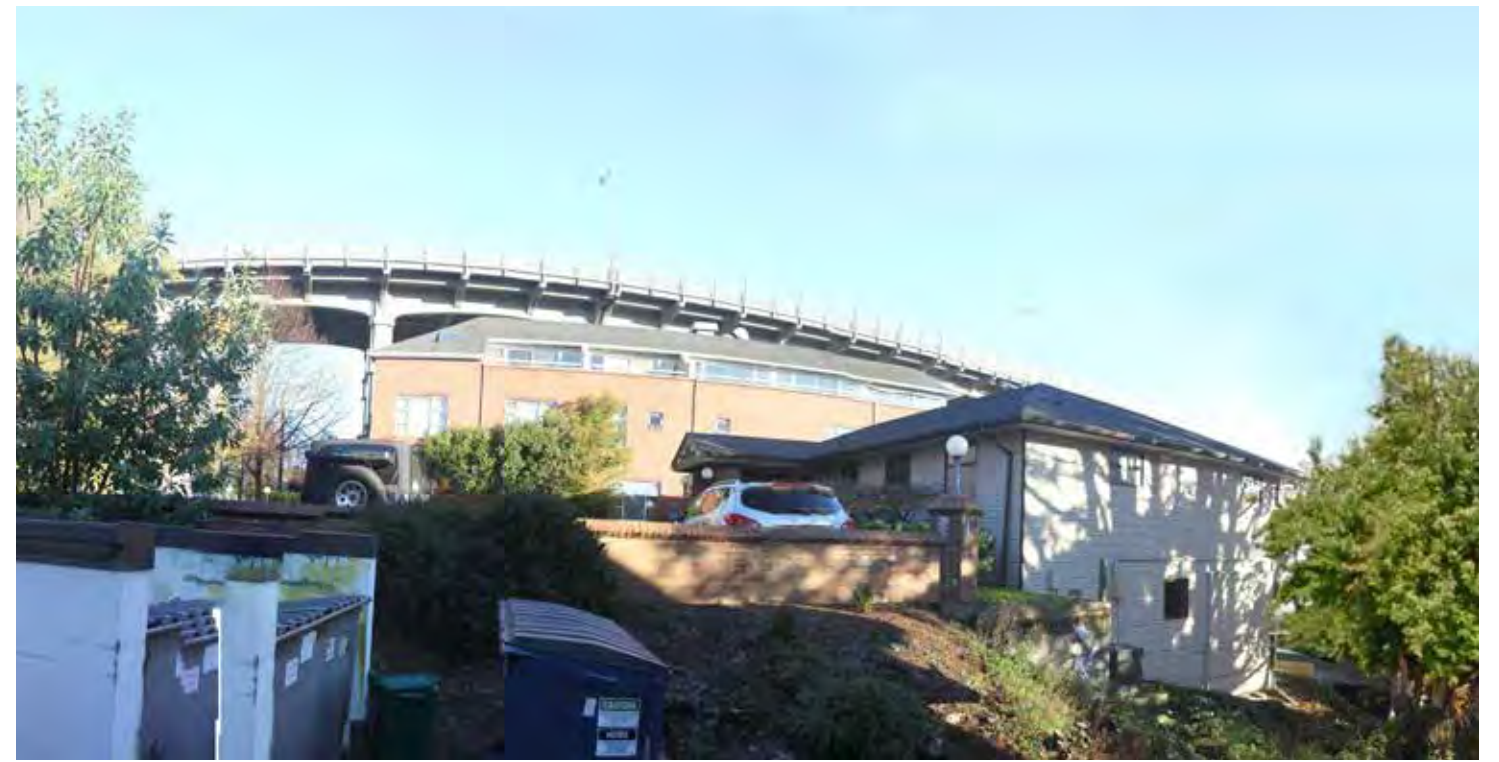
④ West elevation of existing site from Library
