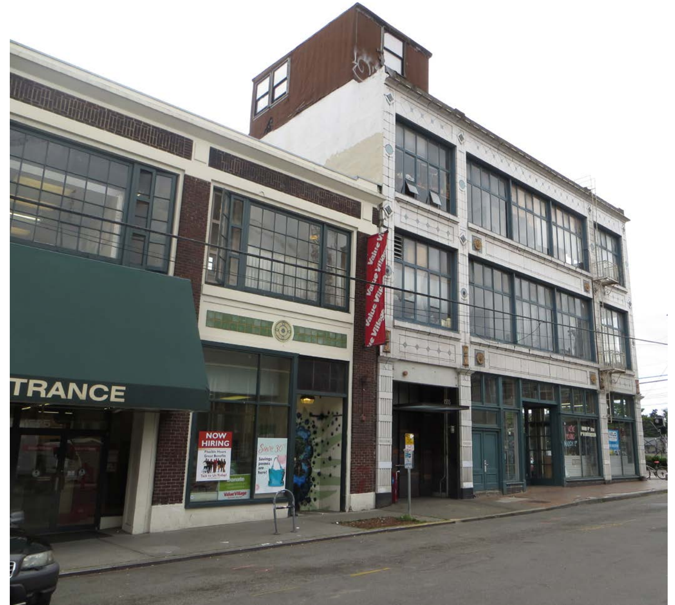
EXTERIOR FACADE WHERE BOCKER/BROWN BUILDINGS ABUT | The second level floorline of the two buildings is very close. A level second floor will not significantly affect the perception of interior volumes.
