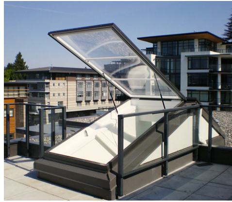
⑧ ROOF HATCH
