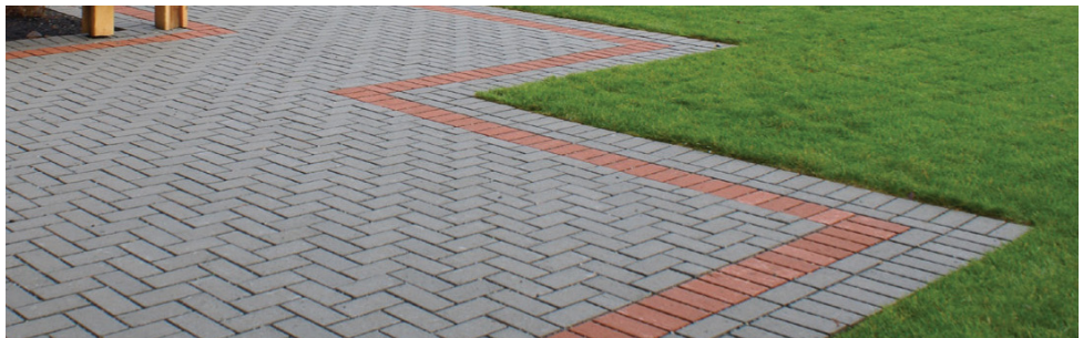
⑦ PATIO PAVING
