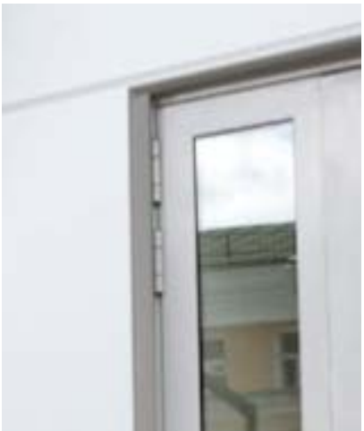
METAL CLADDING AT DOORWAY
