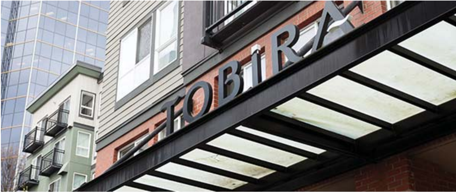
EXAMPLE OF CANOPY MOUNTED LETTERING
