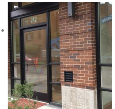
Brick over Concrete (rusticated brickwork)
