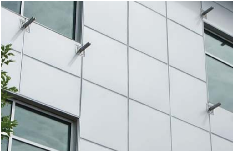
METAL CLADDING AT WINDOWS
