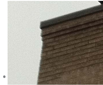
Brick Corbelling and Metal Flashing
