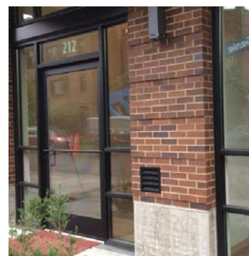
Brick on Concrete
