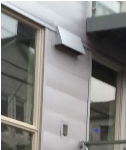
METAL CLADDING WITH VENT
