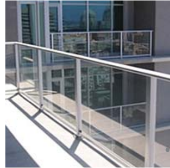
Glass Roof Railing
