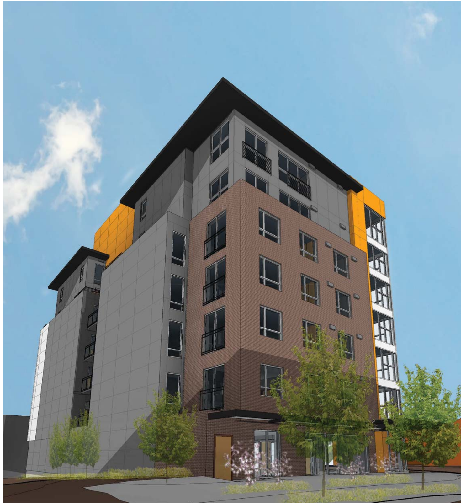
Looking up at the corner of the southwest building
