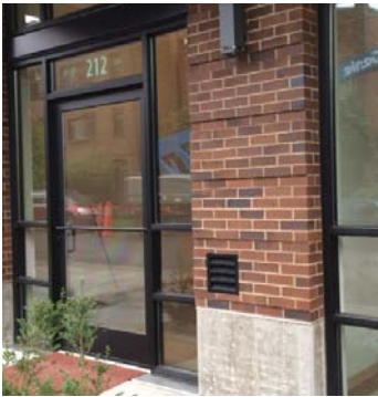
Brick on Concrete
