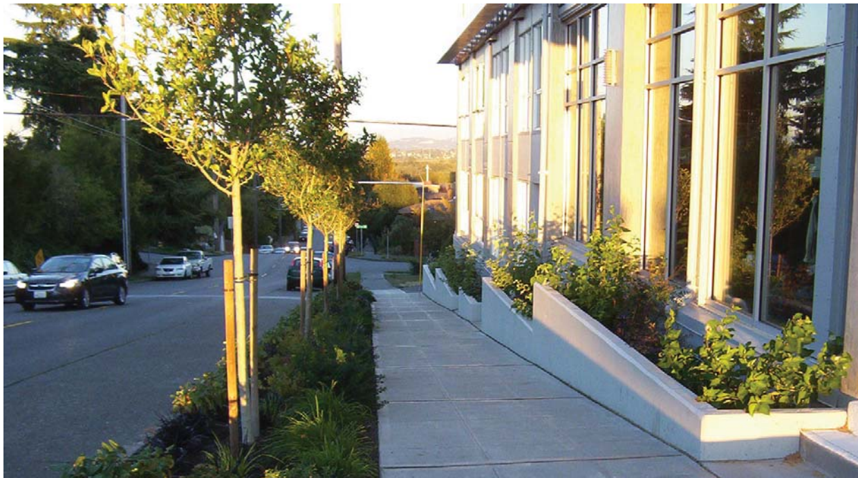
SW OREGON STREET SIDEWALK EAST OF SITE - NOTE : THE PLANTING STRIP IS LESS THAN 4' WIDE AND THE 3' SETBACK IS USED FOR STORMWATER DETENTION AGAINST THE BUILDING
