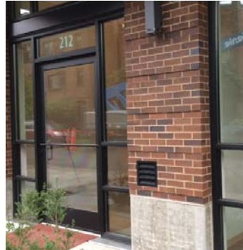
Brick on Concrete
