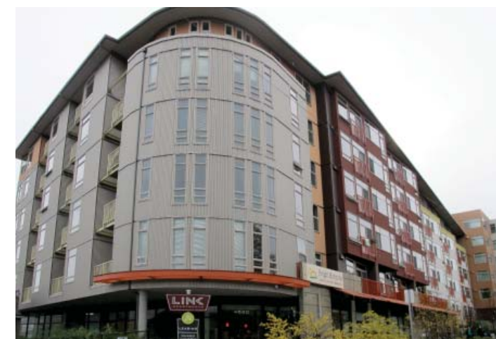
⑪ LINK APARTMENTS
