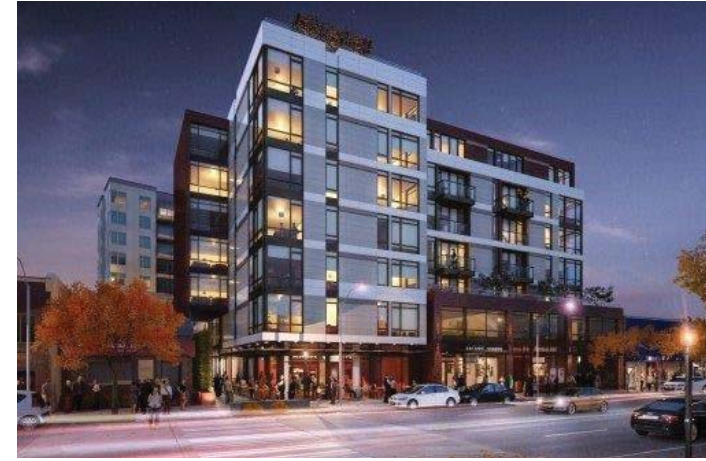
③ 4730 CALIFORNIA (CONSTR)
