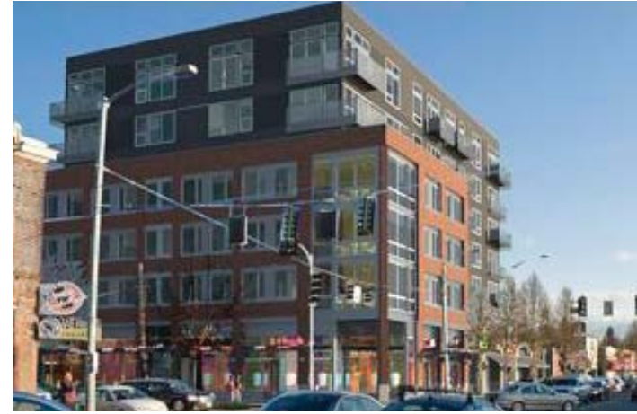
② CONNER BUILDING (CONSTR)
