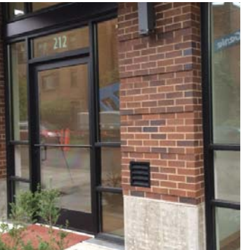
Brick on Concrete
