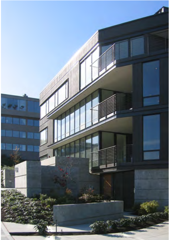
Stadium 302 - Workshop AD
