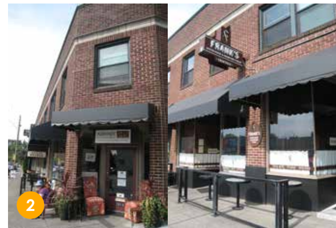
2 Brick facade, corner entry, large storefront windows
