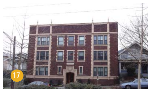
use of brick facade facade broken up by use of trim
