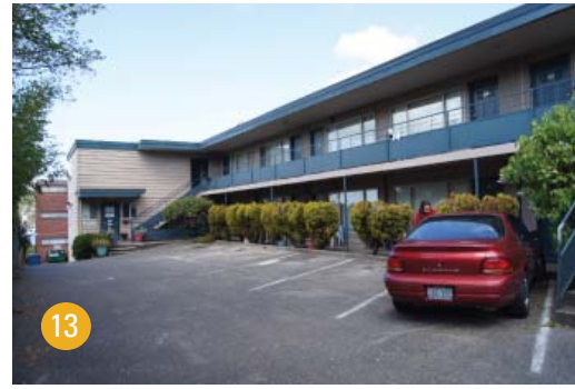
expansive asphalt surface
