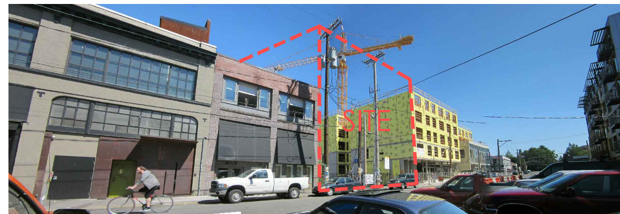
Ⓞ project site- 10th avenue looking south
