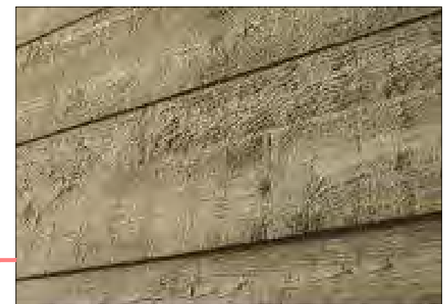
BOARD FORMED CAST-IN-PLACE CONCRETE DURABLE MATERIAL - graffiti-proof "STRONG" DESIGN - adds industrial look at building base
