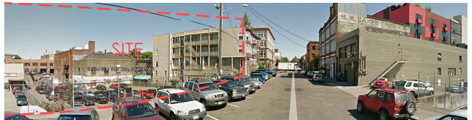
ⓑ PROJECT SITE- 11TH AVENUE LOOKING NORTH
