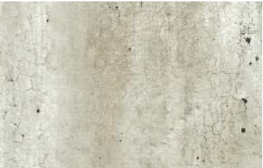
Natural Concrete @ Retaining Walls
