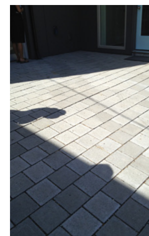
An example of permeable paving from a SFR in Queen Anne. (Playhouse Design Group)
