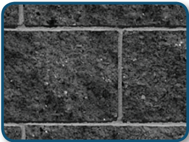
masonry: dark brown roman brick, charcoal split face CMU w/ precast cap
