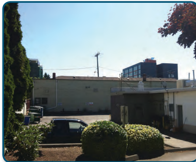
west side view
