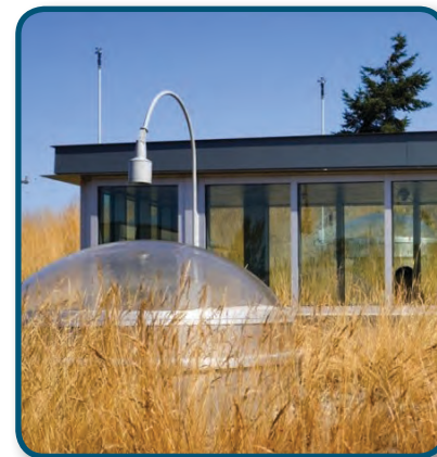
green roof at Ballard Library
