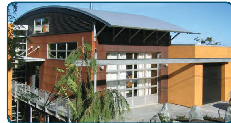
gutters at PLACE architects' Diva make art of the deluge
