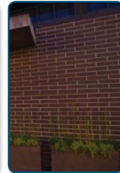
masonry: ground face CMU, split face CMU, roman bricks
