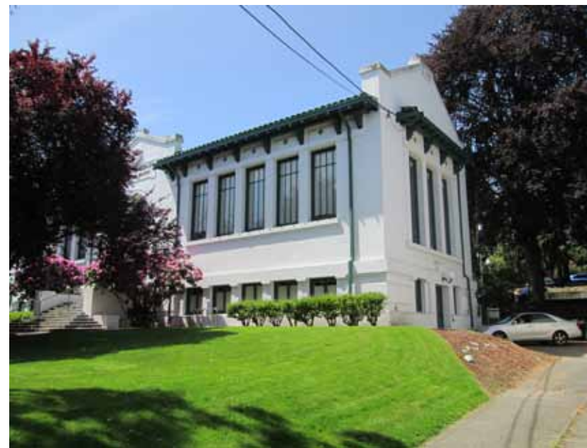
Seattle Public Library, University Branch View of Northeast Corner and Service Drive
