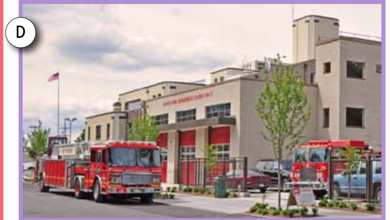
Firestation #17 (Seattle Landmark)
