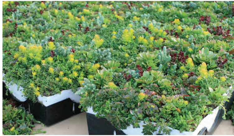
LIVEROOF - GREEN ROOF
