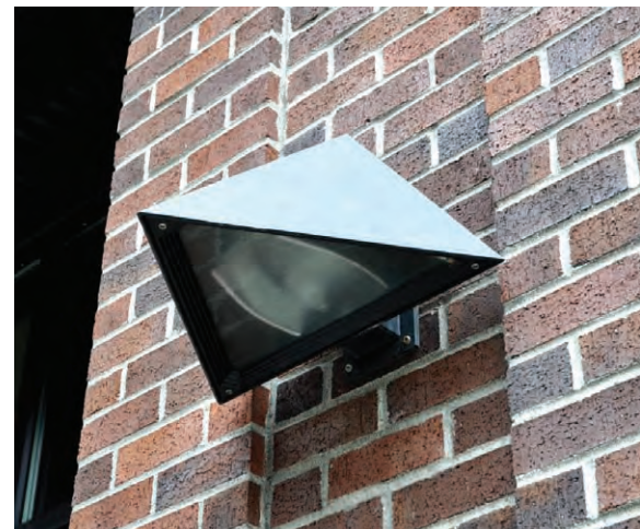
10. GROUND LEVEL SCNCE
