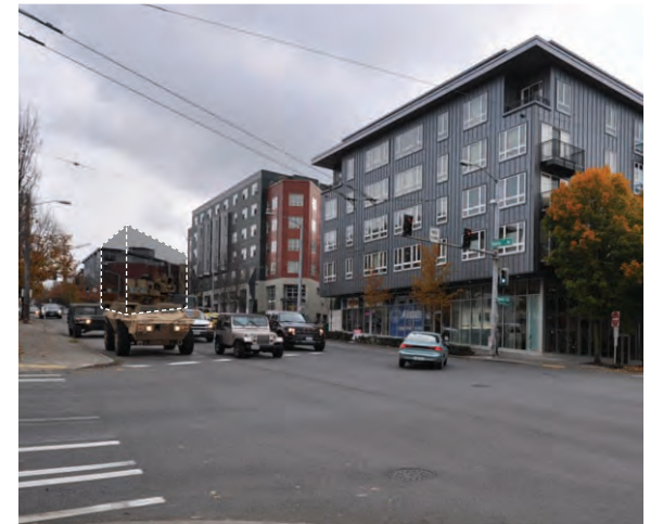
08. SITE | EAST APPROACH FROM DENNY WAY
