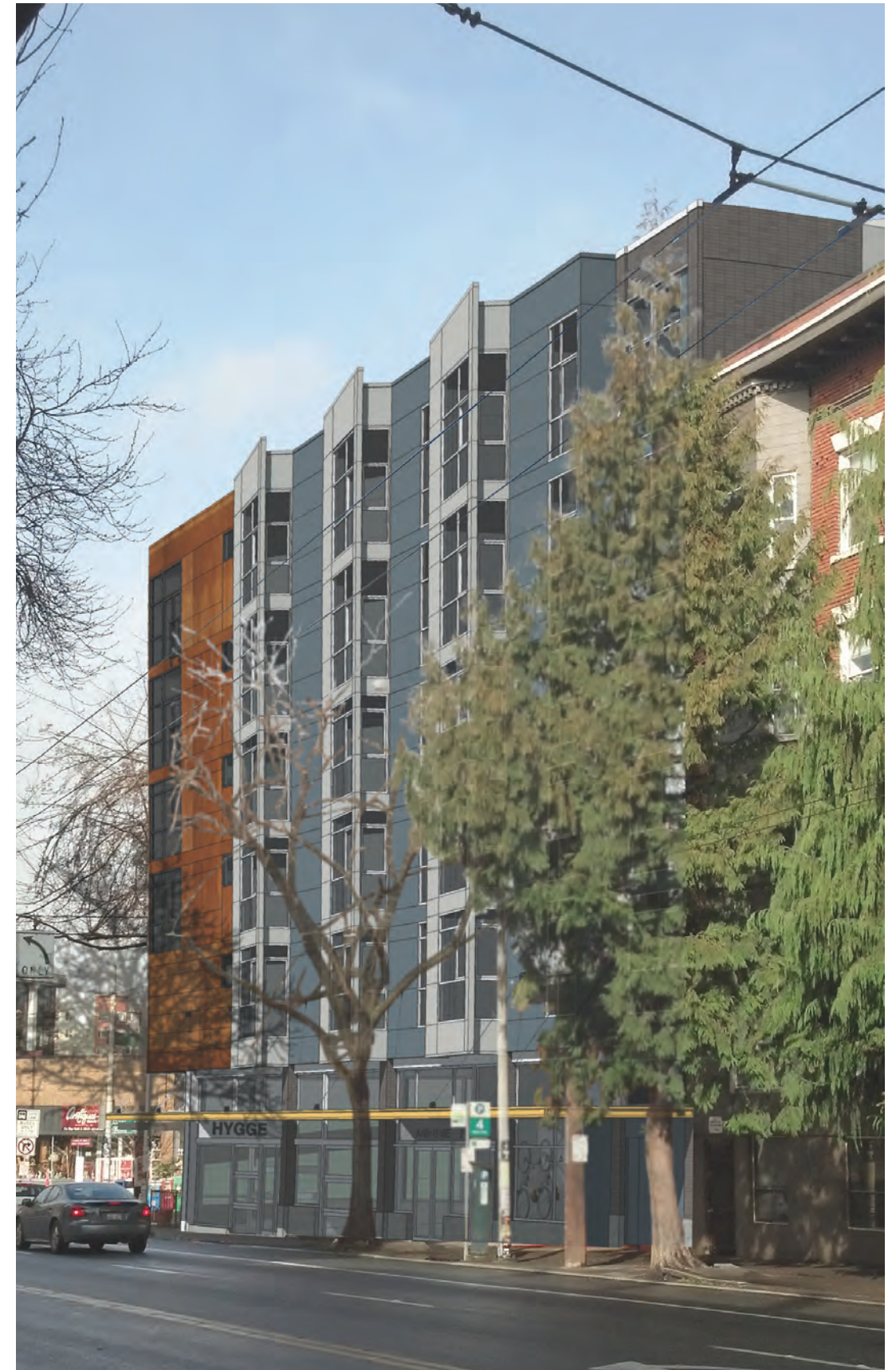
VIEW FROM 1ST AVE LOOKING NW
