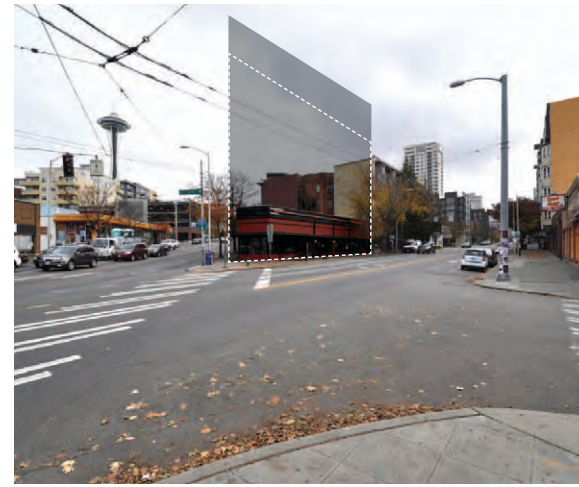
02. SITE | LOOKING EAST DOWN DENNY WAY
