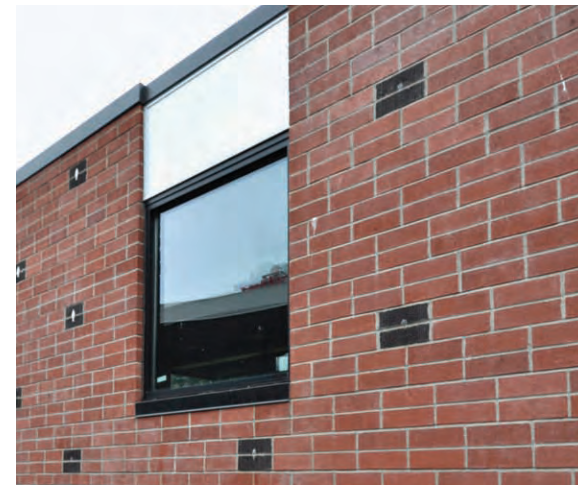
07. VIEW OF BRICK COURSING
