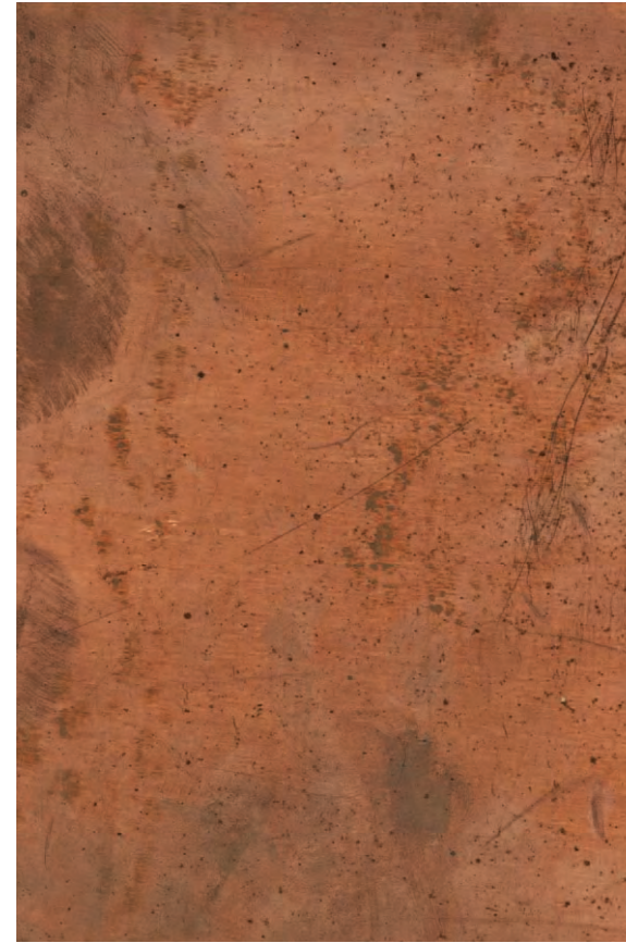
MAIN FIELD CORTEN STEEL SIDING
