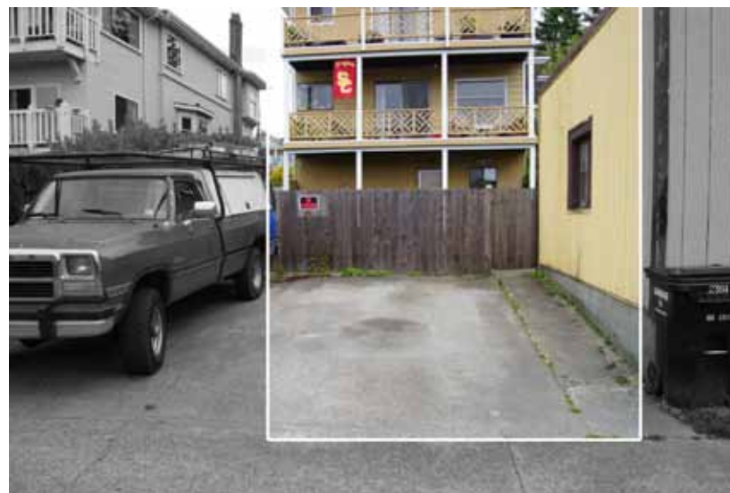
2 view from alley | back facade
