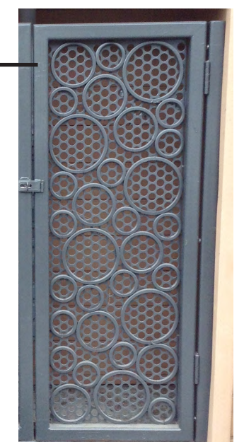
GAS METER SCREENING: PERFORATED METAL PANEL WITH PAINTED METAL BUILDING SIGNAGE AND LOGO DESIGN
