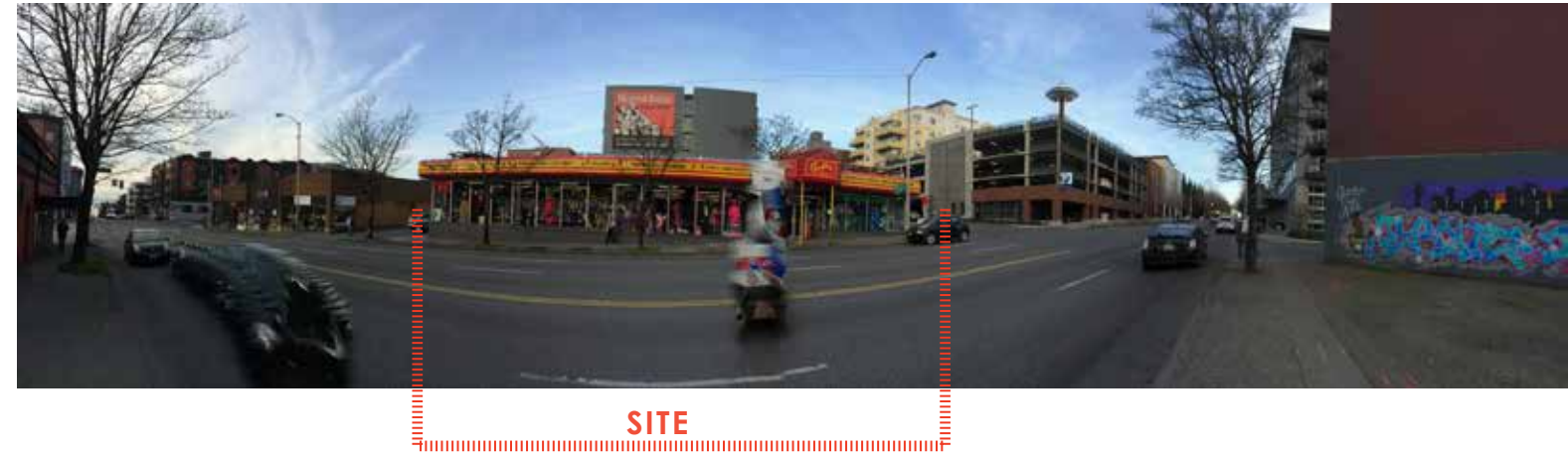
4 View OF site across Denny Way
