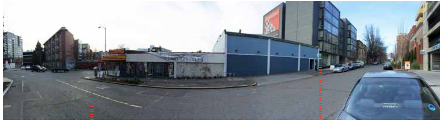
1 View OF site from across Warren Ave. N.
