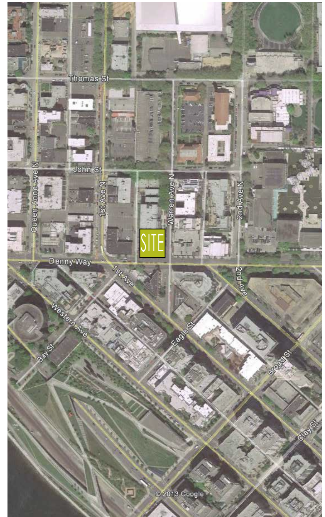
Immediate Location - Aerial Photo
