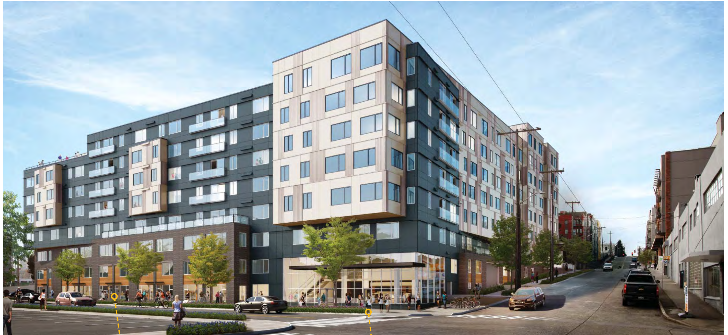
VIEW TO BUILDING AT 8TH & ALOHA
