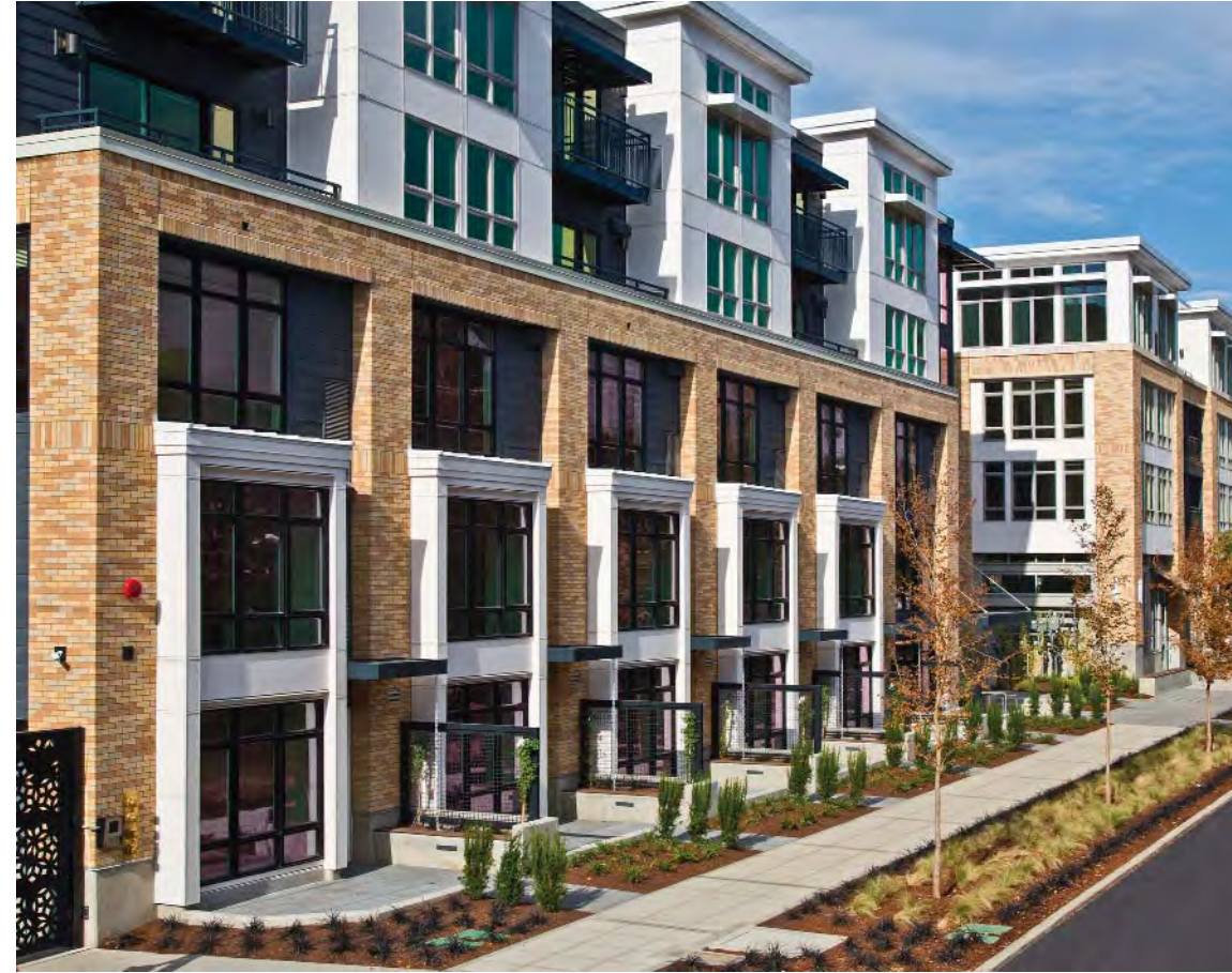
LYRIC APARTMENTS - GRADE LEVEL RESIDENTIAL UNITS
