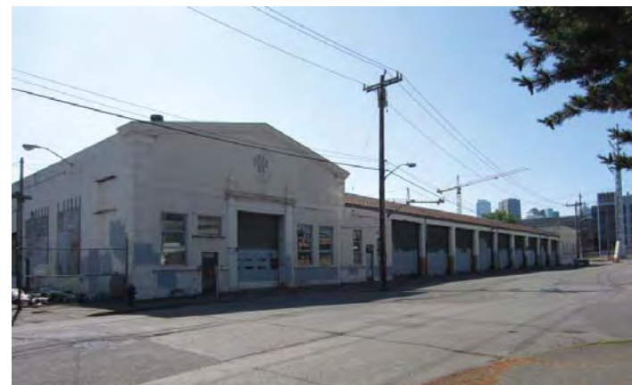
K Puget Sound Power and Light Co. Utilities Building (Seattle Landmark)
