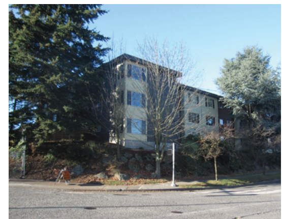
⑤ APARTMENT (NW ON 23RD)
