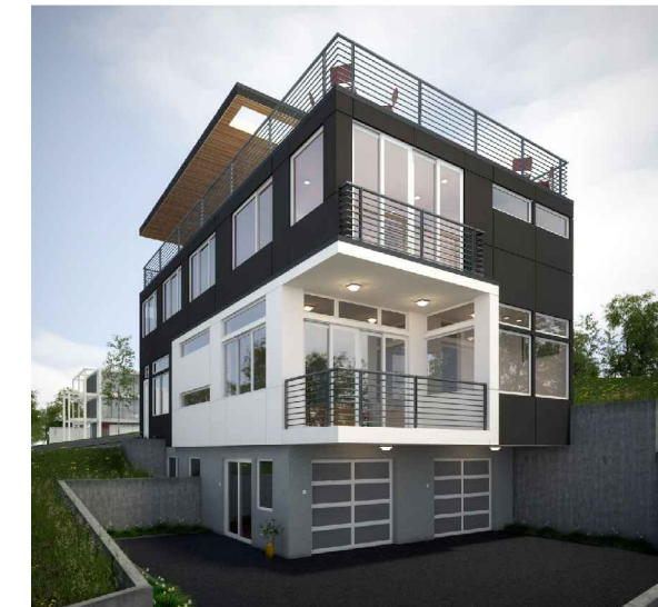
Example of our use of Hardi-Panel & Metal Rail.
