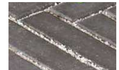
Paving at pedestrian walkways
