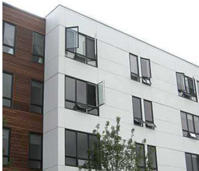
Smooth cement fiber board on body
