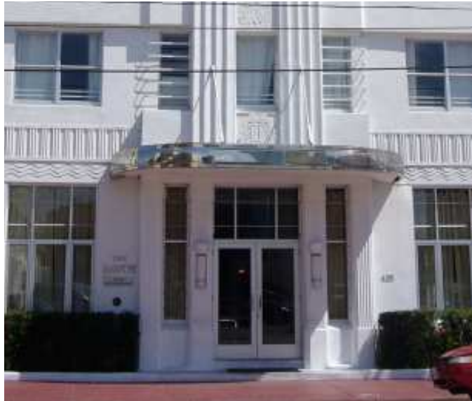
Metal-faced awning above entry
