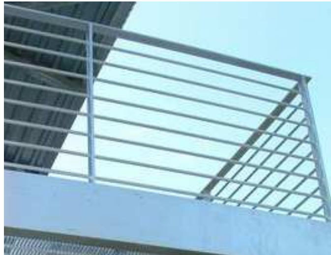
Metal railing and banding at decks
