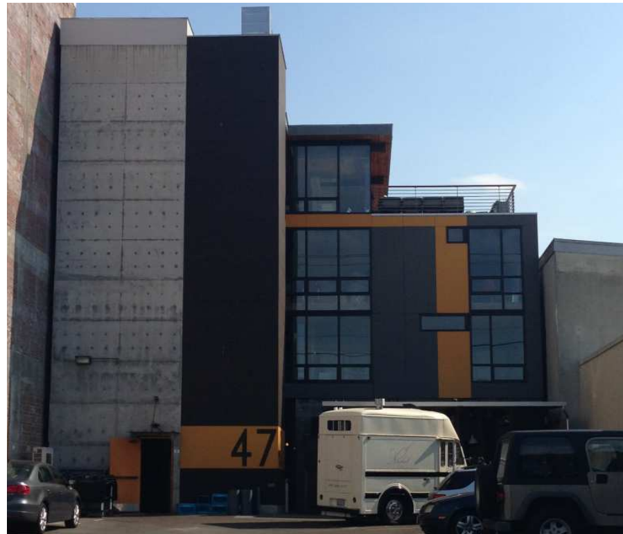
Kolstrand Building, Ballard
