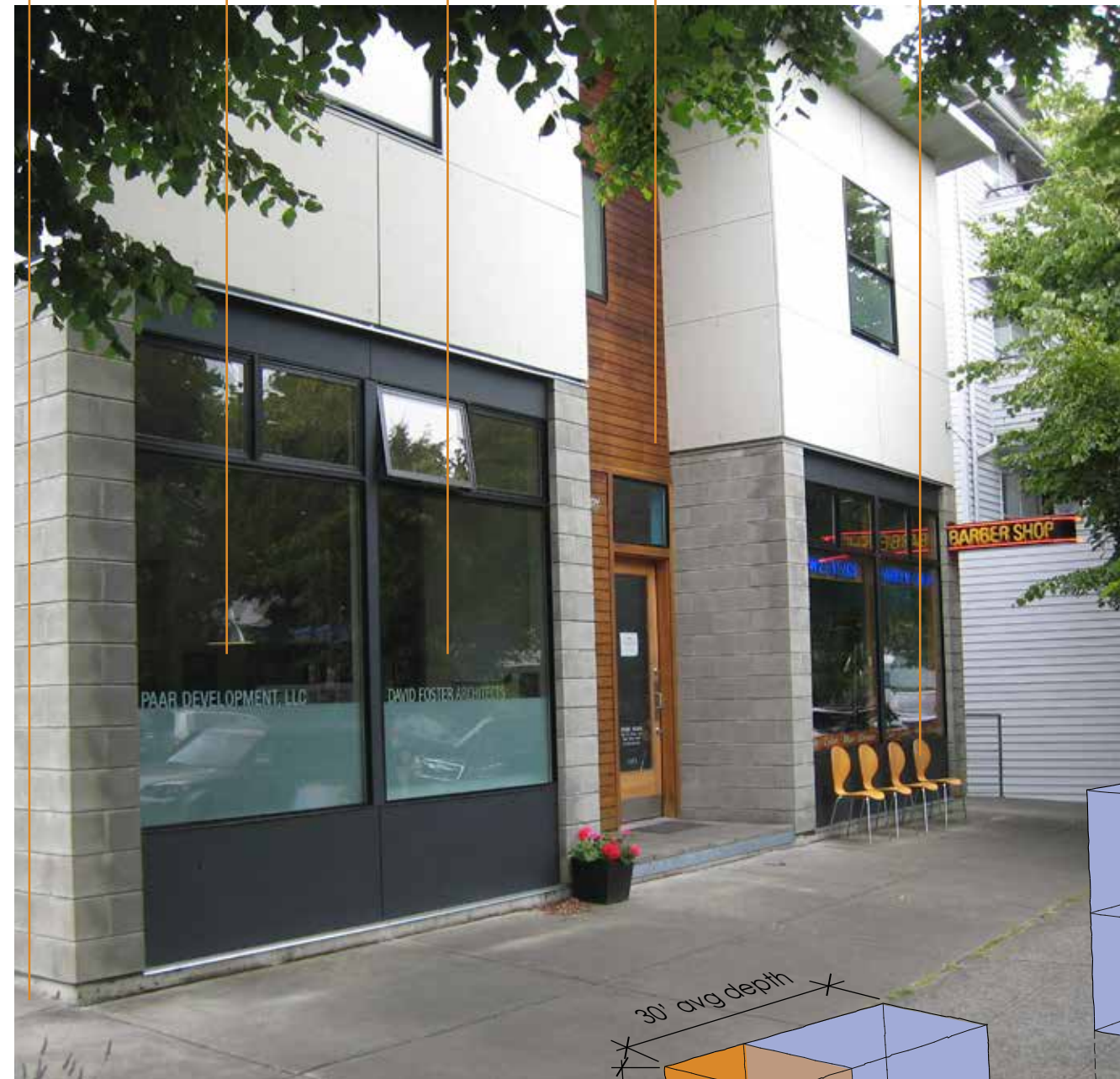
Successful Live-Work on California Ave SW
