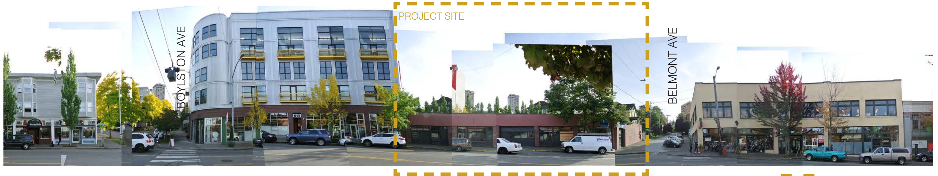
B E. PIKE STREET - LOOKING SOUTH
