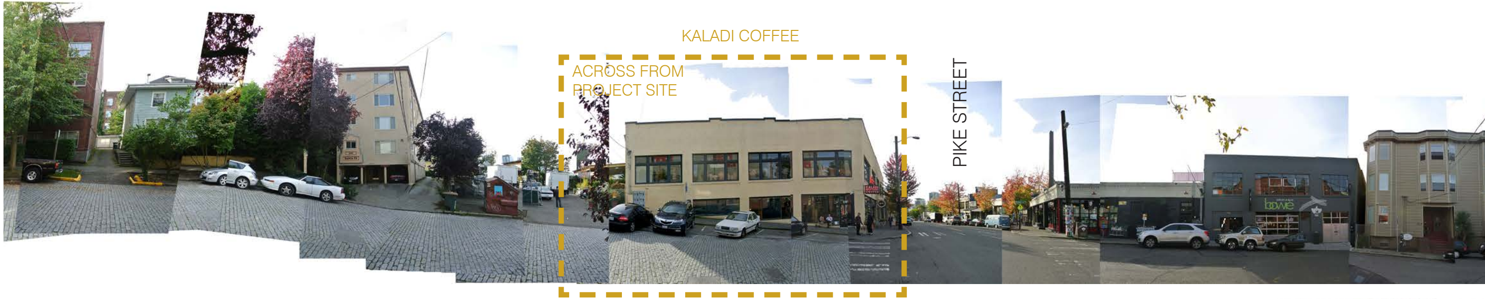
C BELMONT AVE. - LOOKING WEST
