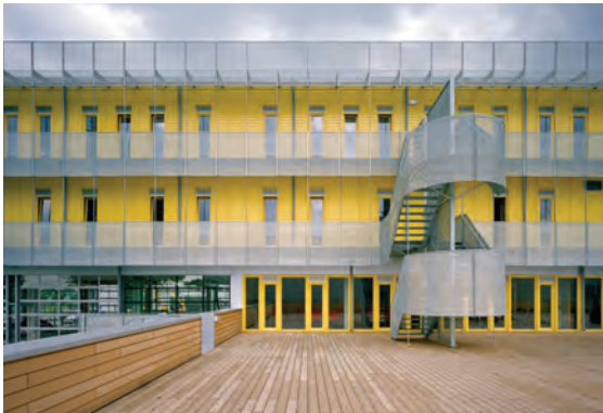
PRECEDENT IMAGES AND SKETCH STUDIES FOR PAINTED STEEL EXTERIOR CIRCULATION ELEMENTS INCLUDING STAIRS, EGRESS BALCONIES AND CANOPIES.
