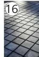
16 PERVIOUS CONCRETE PAVERS - WALKWAY
