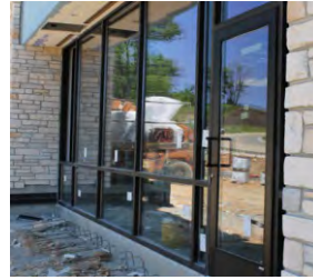
ALUMINUM STOREFRONT SYSTEM, PAINT TBD
