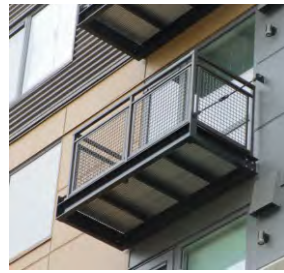
PAINTED STEEL BOLT-ON BALCONY COLOR: SEALSKIN
