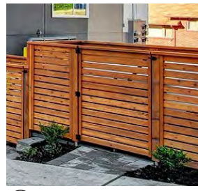
HORIZONTAL CEDAR WOOD GARBAGE/RECYCLE SCREENING
