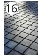
16 PERVIOUS CONCRETE PAVERS - WALKWAY
