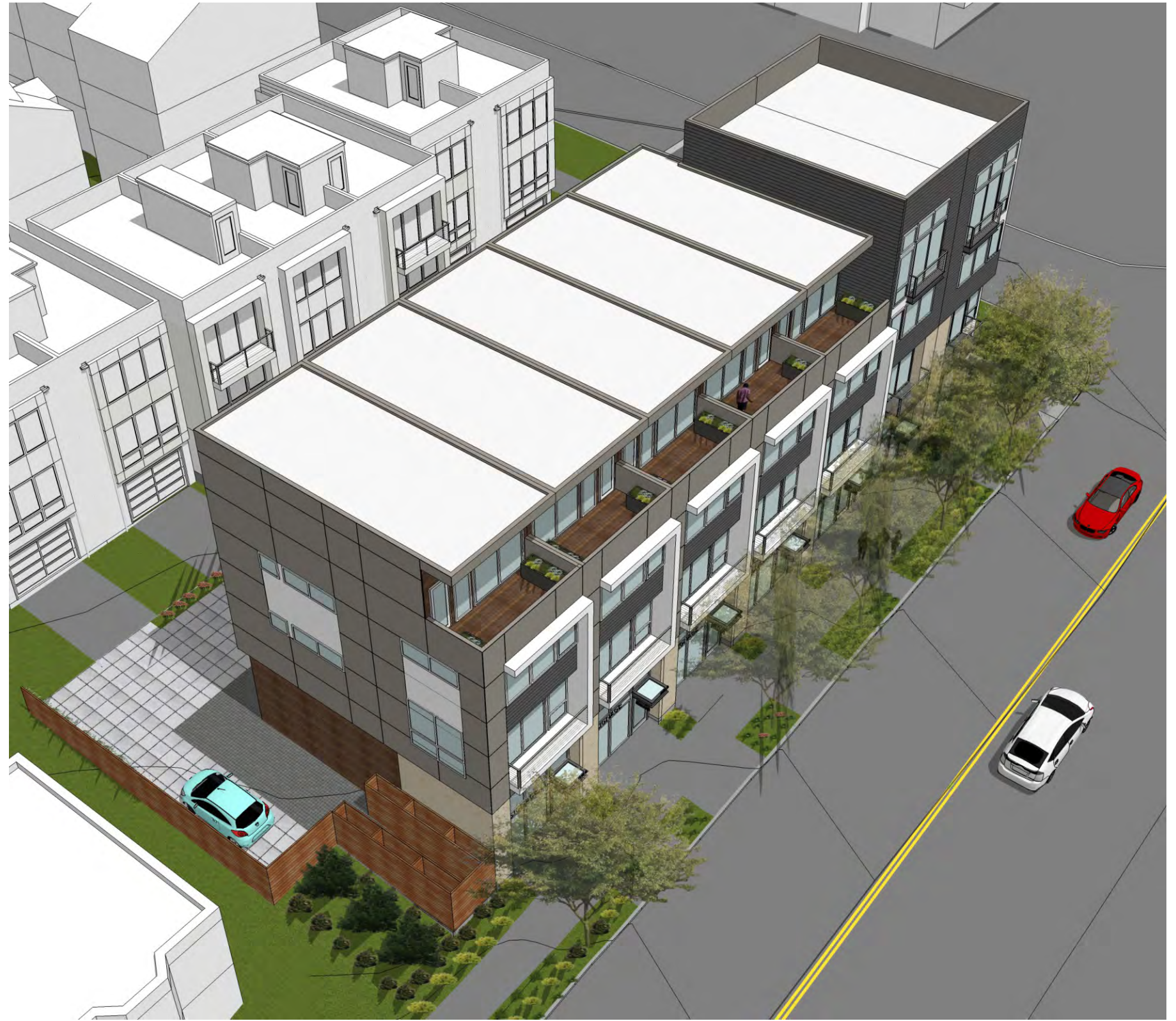
OVERHEAD VIEW LOOKING NORTHEAST
