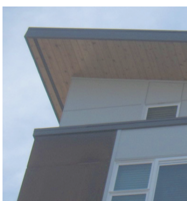
Large overhang, plain soffit
