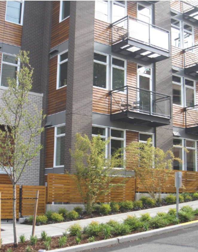
MASONRY WITH INFILL PANELS
