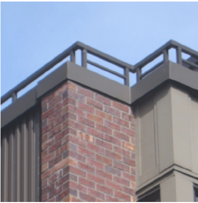
Parapet with partial railing
