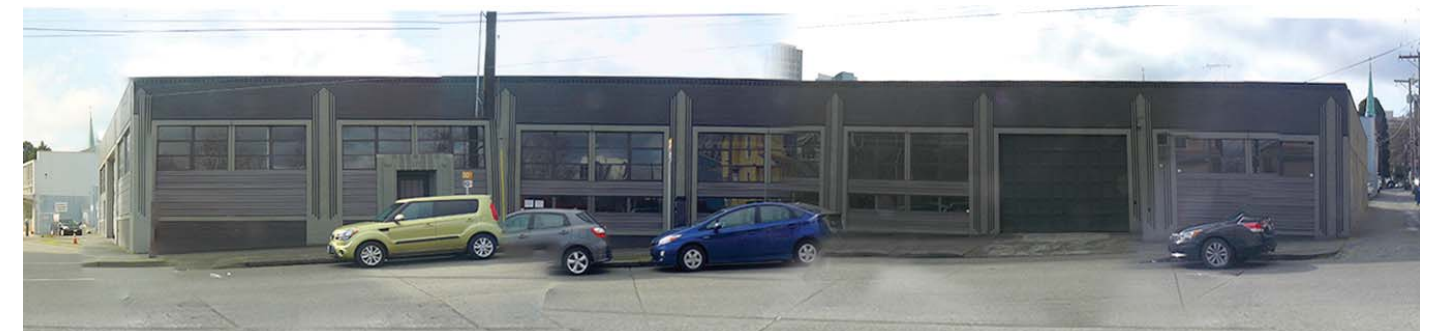
C View looking south from Thomas St.
